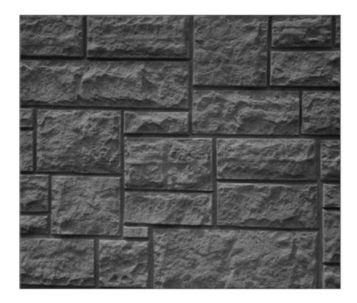
All texture is to be in addition to the nominal thickness of each element within tolerances. Maximum relief of the textured surface shall be 1<sup>1</sup>/<sub>4</sub> inch or less.
